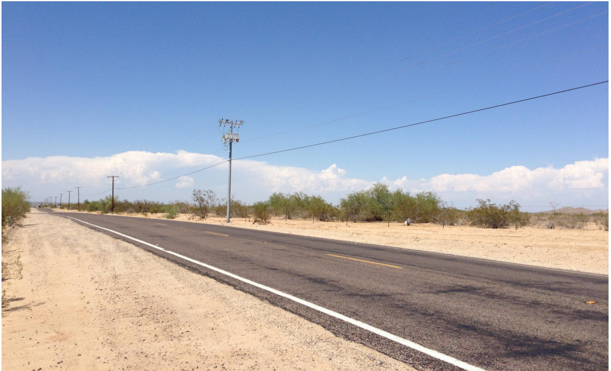
Looking at Property Frontage Along Tuthill
